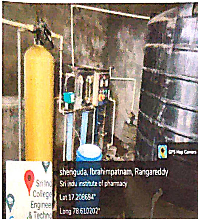
Recycling waste water through RO Plant and treated water storage tank
