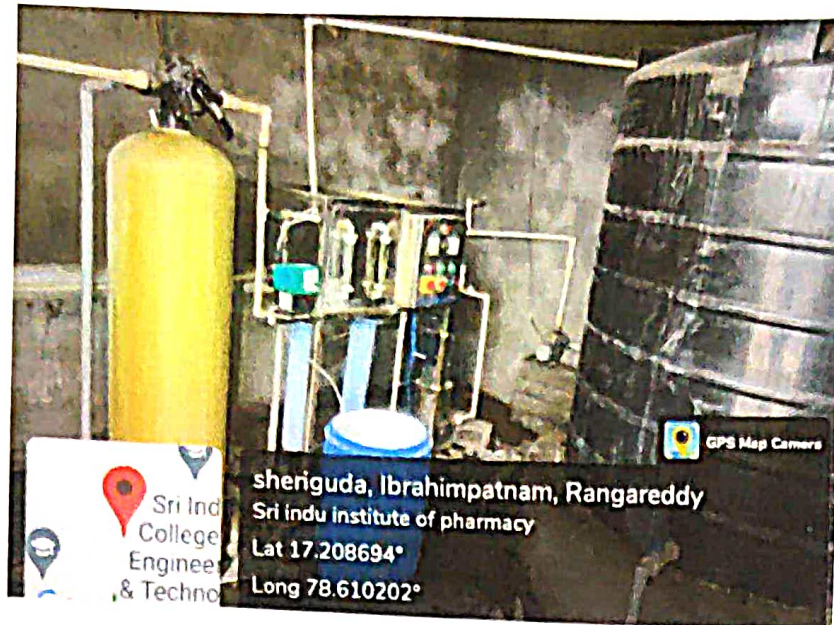
Recycling waste water through RO Plant
